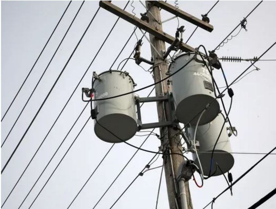
Utility pole with power lines and transformers.
