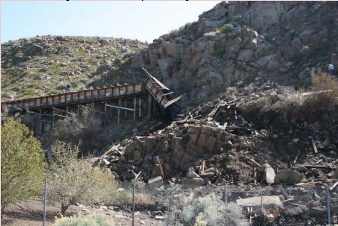
Rock fall damage to water flume
