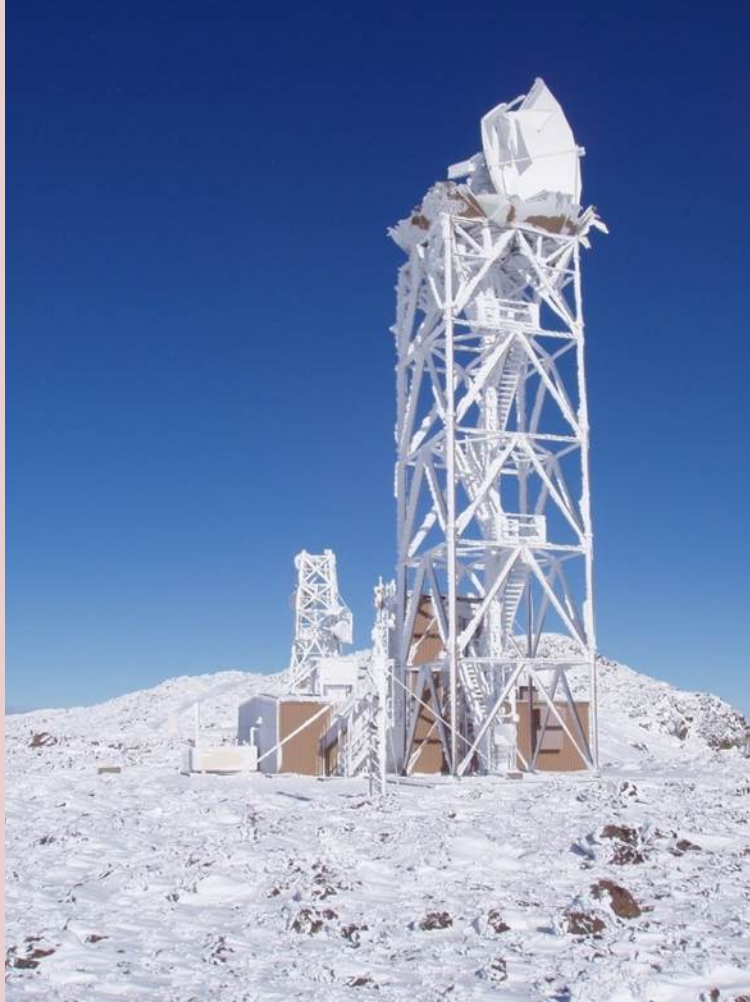
Figure 4-4 NWS Reno Radar Damage from Wind (December 2008)
