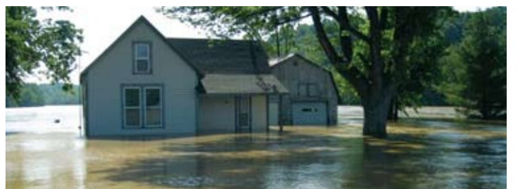
A home that was inundated by the floods.
