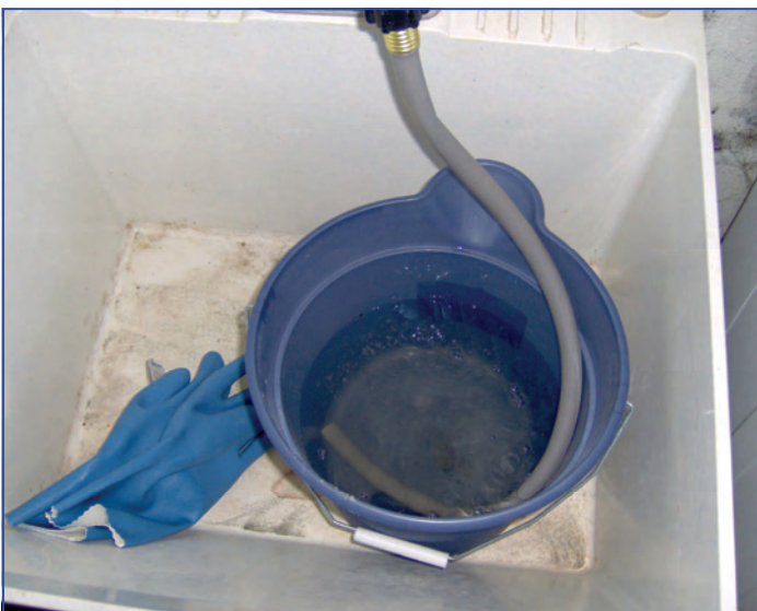
Hose connected to the hot water faucet in a laundry room sink. The bleach solution is being siphoned into the household hot water system.
