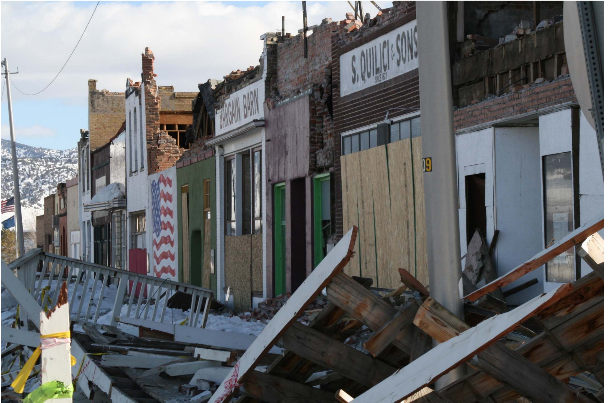
2008 Wells, Nevada Earthquake
