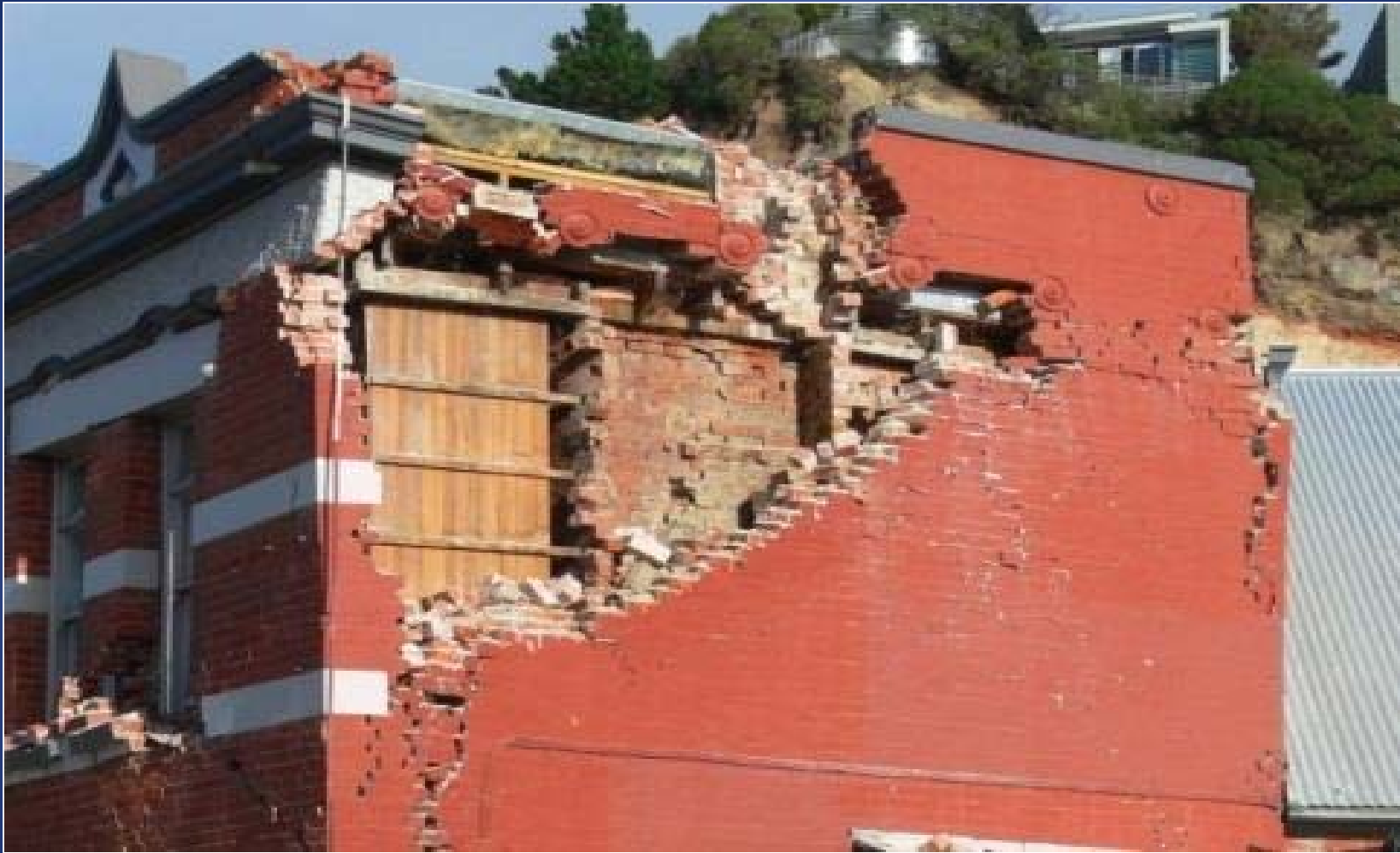
June 13, 2011 Magnitude 5.5 and 6.0 earthquakes 3 mi (5 km) away
