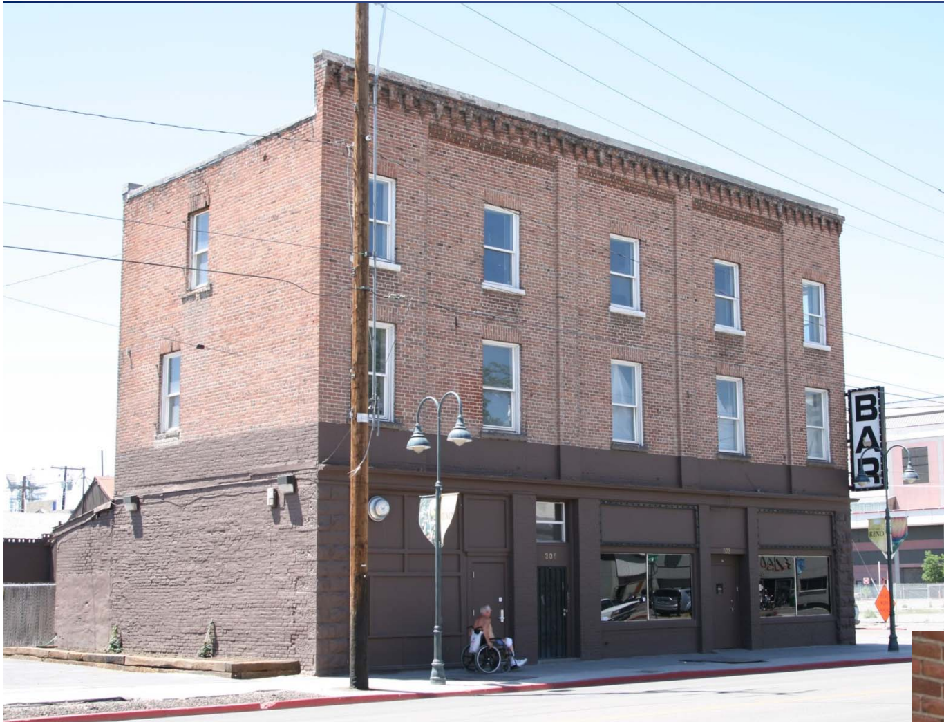
Three-story URMB with parapet and some earthquake cracks; occupancy is variable
