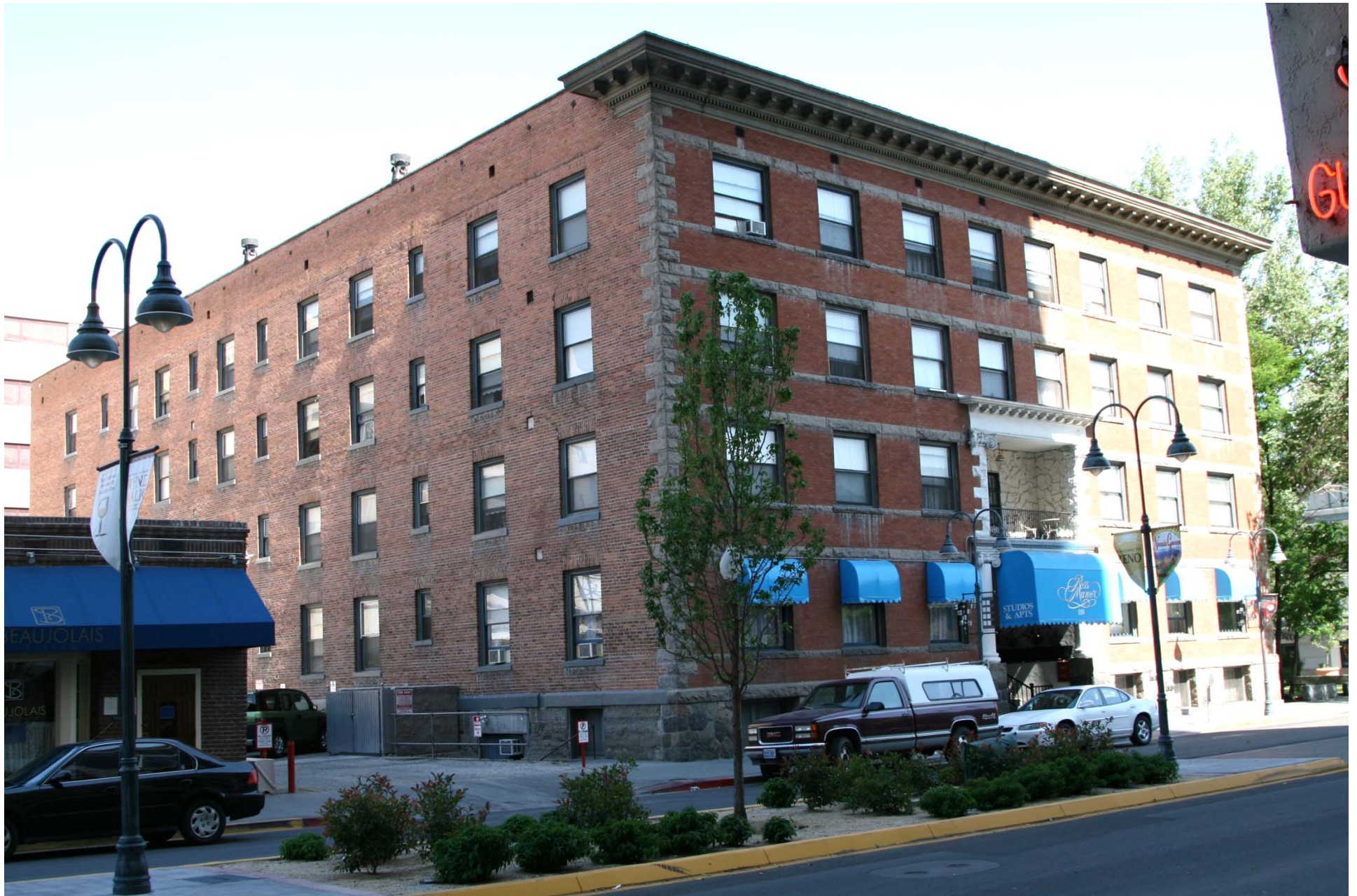
Commercial five-story apartment building; continuous high occupancy
