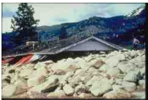
Figure 3-24. Photo of the aftermath of Slide Mountain landslide/Ophir Creek debris flow from NOAA
