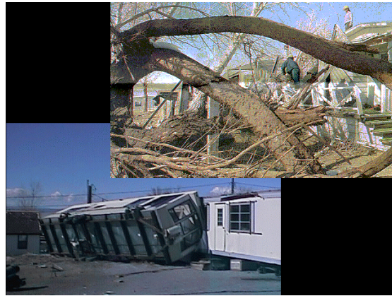
Figure 3-34. Windstorm damage in Gabbs, Nevada, 1998. Photo courtesy of NOAA.
