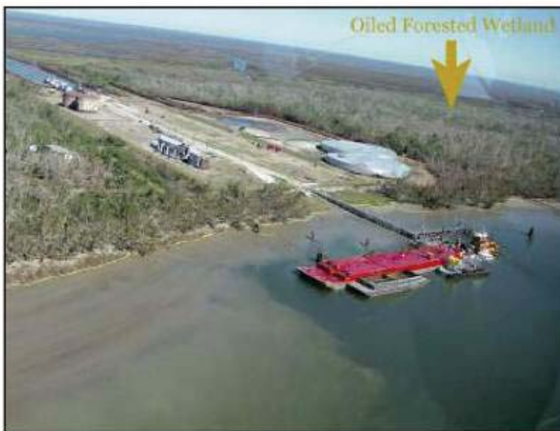
Figure 2: Oil from damaged tanks was moved by hurricane forces into impassable forested wetlands. USCG photo.
